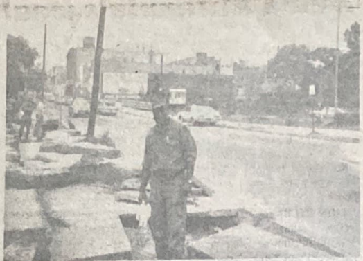
STRONG WATER currents buckled concrete sidewalks on some Chester streets. Hardest hit area was 'Holy City' — a white residential area whose residents have prevented Blacks from buying there.
