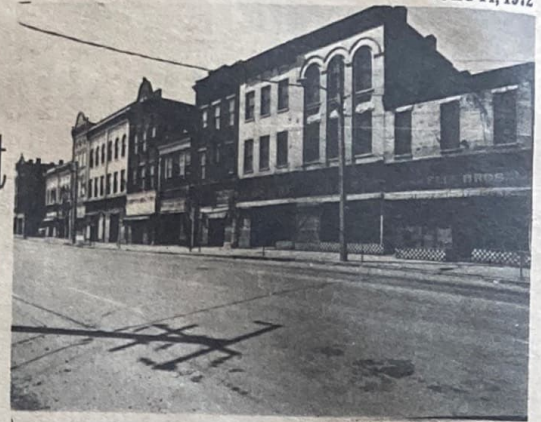
WHOLE BLOCKS of businesses were forced to discontinue operation while hundreds of homes were destroyed by vicious floods. All - Black community of Fulton was hardest hit.
